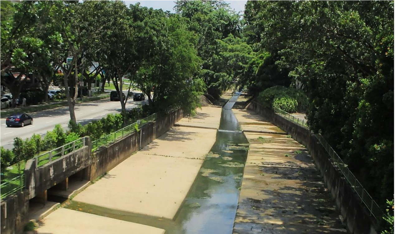
Fig. 298. Looking upstream. Note the expansion needed after the canal was originally constructed to cope with increased volume of water due to rapid urbanisation of the steep valley sides. (Photograph by: A. Gupta).
