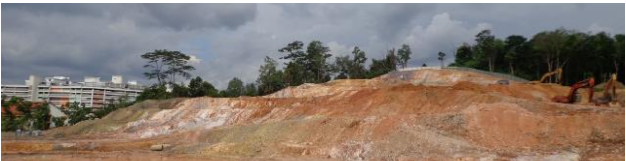
Fig. 275. View to the northeast of the excavations between Bukit Batok West Avenue 2 and Bukit Batok Road. Note that the clay-dominated slope has been cut back to 20°. (Photograph by: G. J. H. Oliver in 2016).
