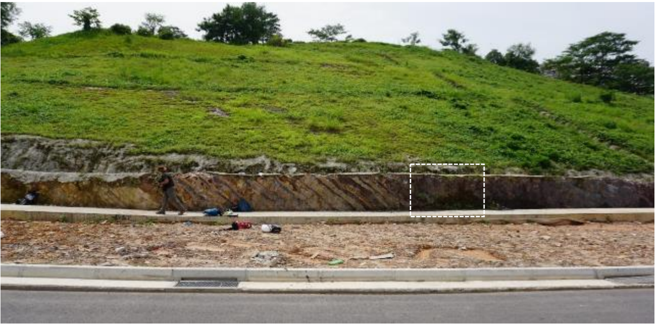
Fig. 268. Location 2: Road cut at the base of the red and purple beds mapped in Fig. 265, looking southeast. (Photograph by: G. J. H. Oliver).
