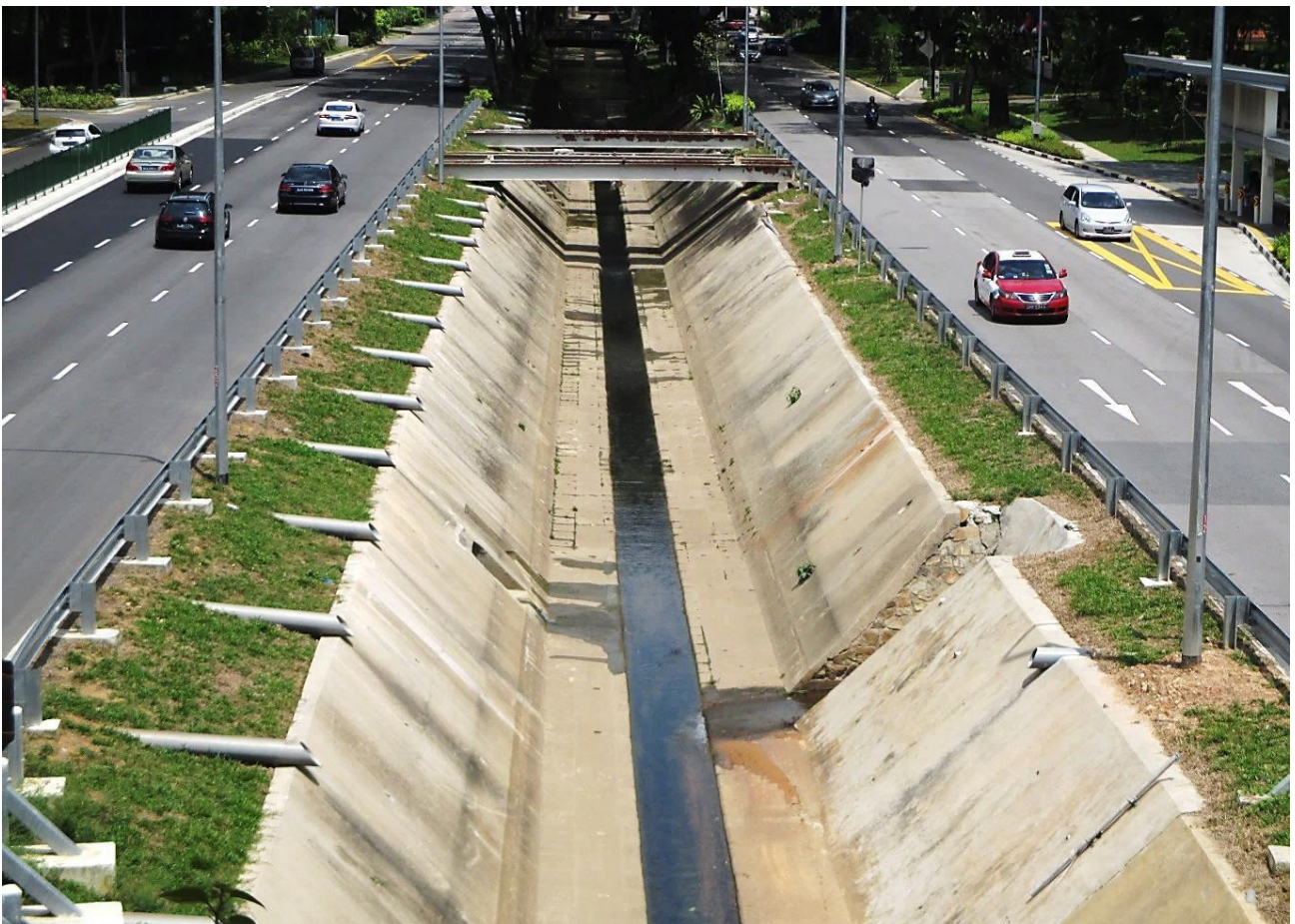
Fig. 294. The concrete-lined upper Bukit Timah Canal as seen from the new bridge near the Albert Park MRT station. Note the shape of the entire canal and the low-flow channel in the bottom. Storm drainage from side valleys reach the canal rapidly after a rainstorm. The arterial roads of Bukit Timah and Dunearn occur on floodplains on either side of the canal. (Photograph by: A. Gupta).
